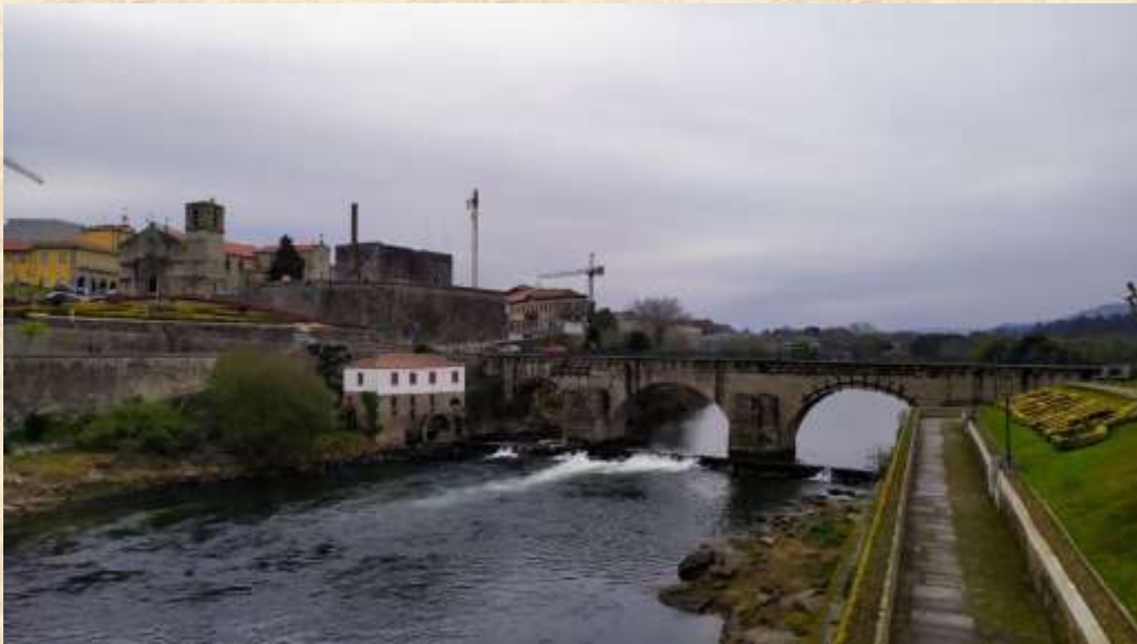
A medieval bridge over the river Cavado.
